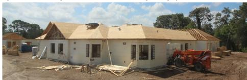
The unique part of these projects is the foam block construction. It is similar to building a very large cooler. The foam block has a center cavity into which concrete is poured. A fire lid is constructed directly to the truss system and, once all work is completed in the attic, insulation is then blown into the attic, making for a very energy efficient system.
